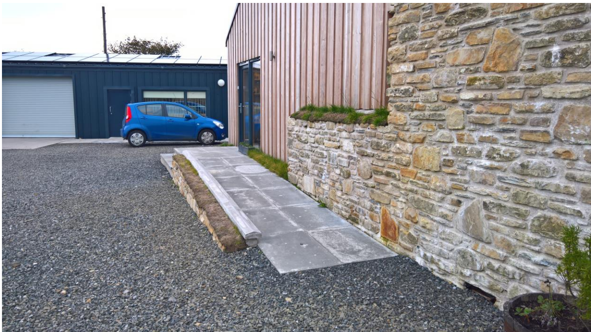
Ramp access to the Main Entrance to the Visitor Centre.
